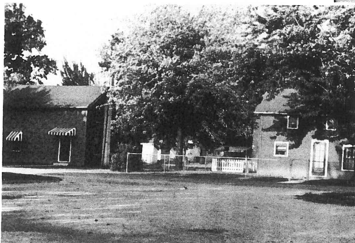
In the early days, these two houses were one large building serving as a boarding house during shipbuilding industry at Shepherdsville.
