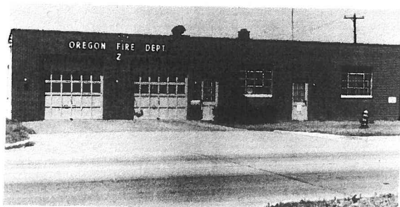
Fire Station No. 2 on Wheeling near Pickle.
